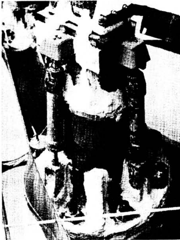
Figure 18.- Hold-down post M-3 prior to launch (STS-3).
